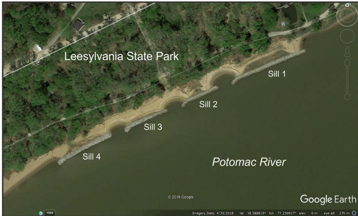
Figure 6. Google Earth image showing the installation of all four sills as designed. As of the photo date, sills 1 and 2 had been in place for about 1.75 years. The remainder of sill 3 and sill 4 had just recently been installed.
