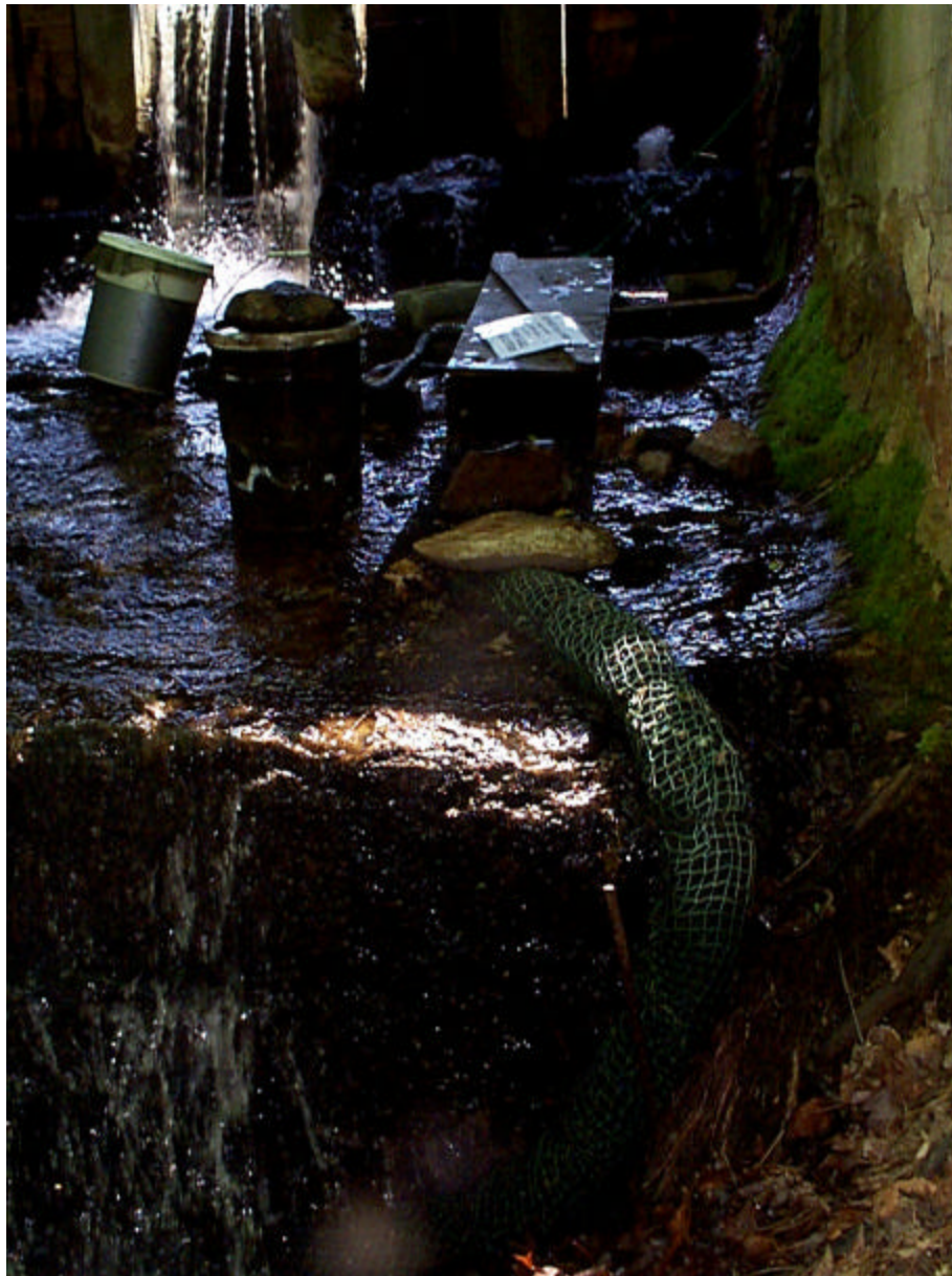
Figure 3. The Irish ramp at Clark's Millpond (Coan River). The green tube in the foreground is the modified ramp extension.
