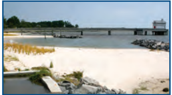
New elevated concrete pier and stone breakwaters minimized damage to the VIMS shoreline during Hurricane Irene.
