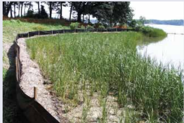
Figure 12. Newly planted marsh with fiber logs allow plants to establish root system and stabilize shoreline. Source: VIMS, 2006.
