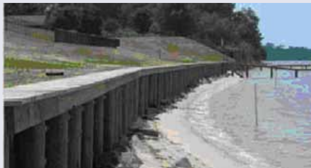
Figure 9. Armored shoreline. Source: VA CZM, n.d.
