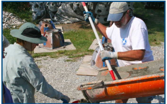
Pouring Concrete: VIMS alumnus Tommy Leggett and some volunteers use marine-safe cement to create reef-balls for oyster restoration. Photo by David Malmquist
