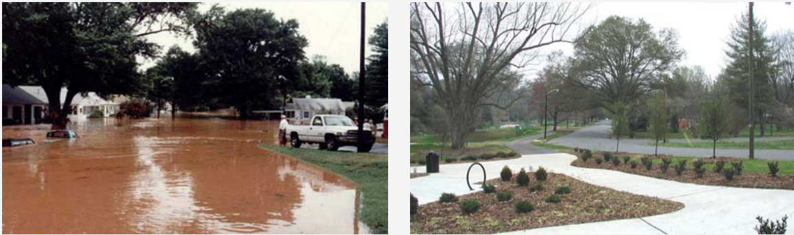
Westfield Road in Charlotte, North Carolina, during a flood on Aug. 4, 2011, left, and after Mecklenburg County's Floodplain Buyout Program bought and removed homes on the street and converted the land into greenspace, right, which helps absorb excess water and provides environmental and recreational co-benefits. Charlotte-Mecklenburg Storm Water Services
